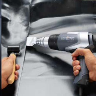
▲ Welding pond liner HG 2320 E
