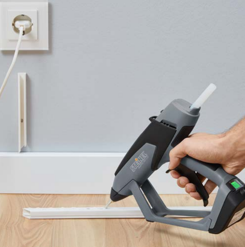
▲ Affixing Permanently mounting cable ducts/trunking with acrylate-based adhesive.
